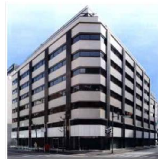
Toranomon 5 Mori Building
